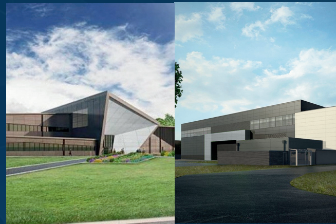
Defence & Secure Facilities
